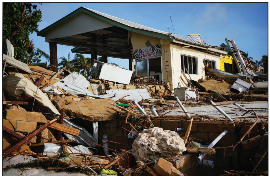
Vakaloa Beach Resort, Kanokupolu. Damage primarily from TC Harold Storm surge. Picture by Henry Todd
